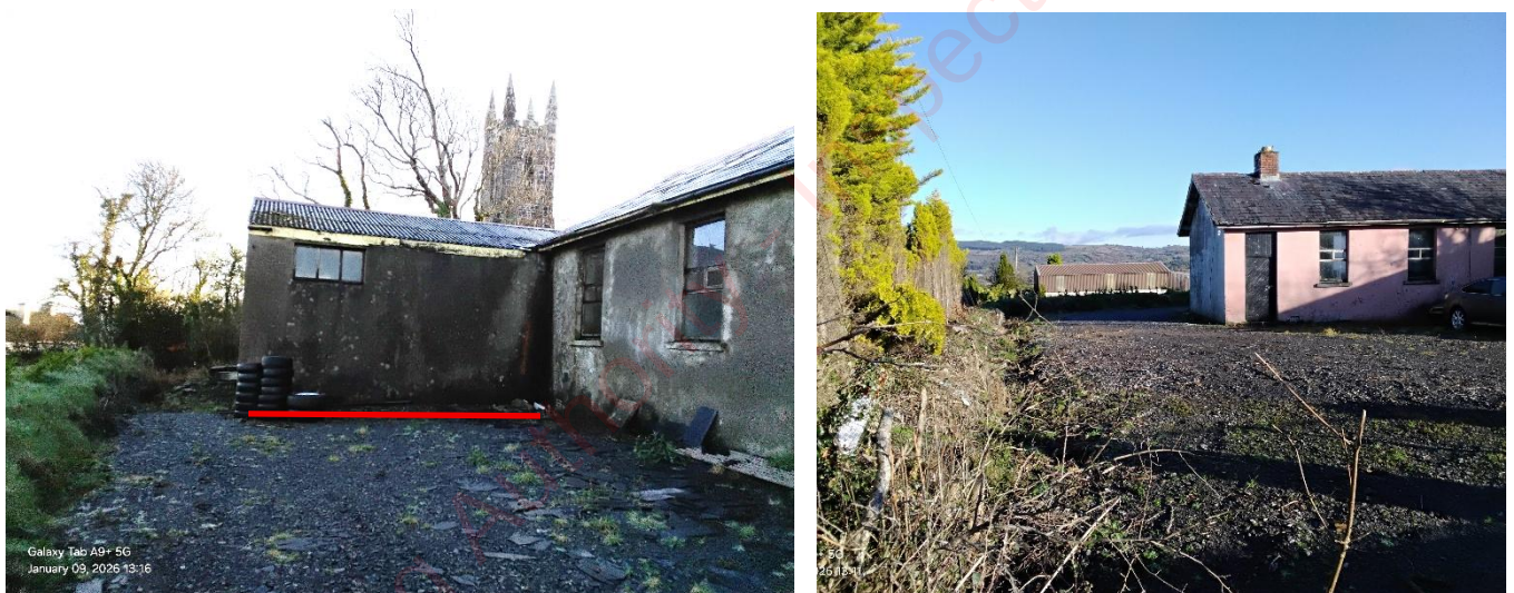
Fig. 3 Location of proposed extension and site viewed from the western boundary
