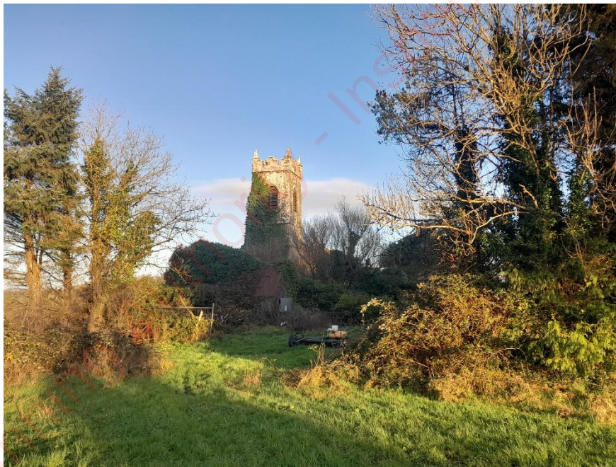
Fig. 3 – View of church (LE015-111001)
